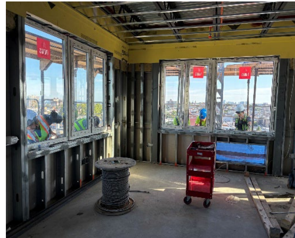
Window Installation on the 13 th Floor
