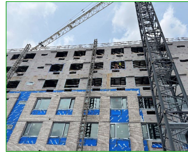
Brick Installation up to the 13 th Floor
