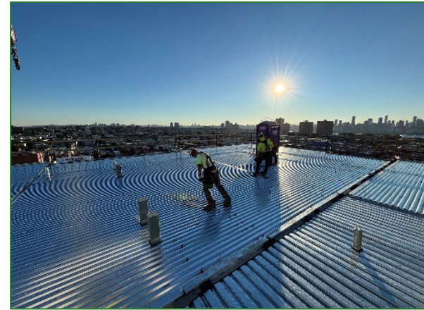
Decking Installation on the 14 th Floor
