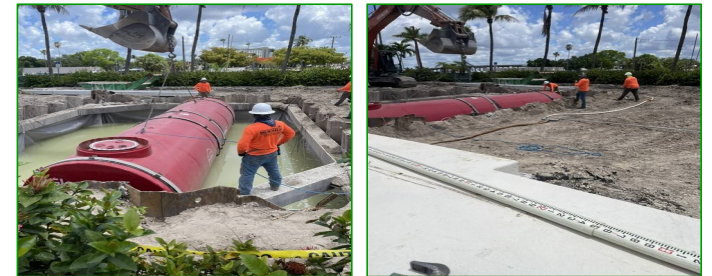
Fuel Tank Installation
