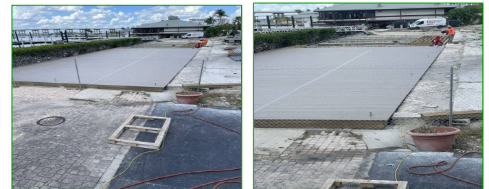
Progress on the Marina Deck
